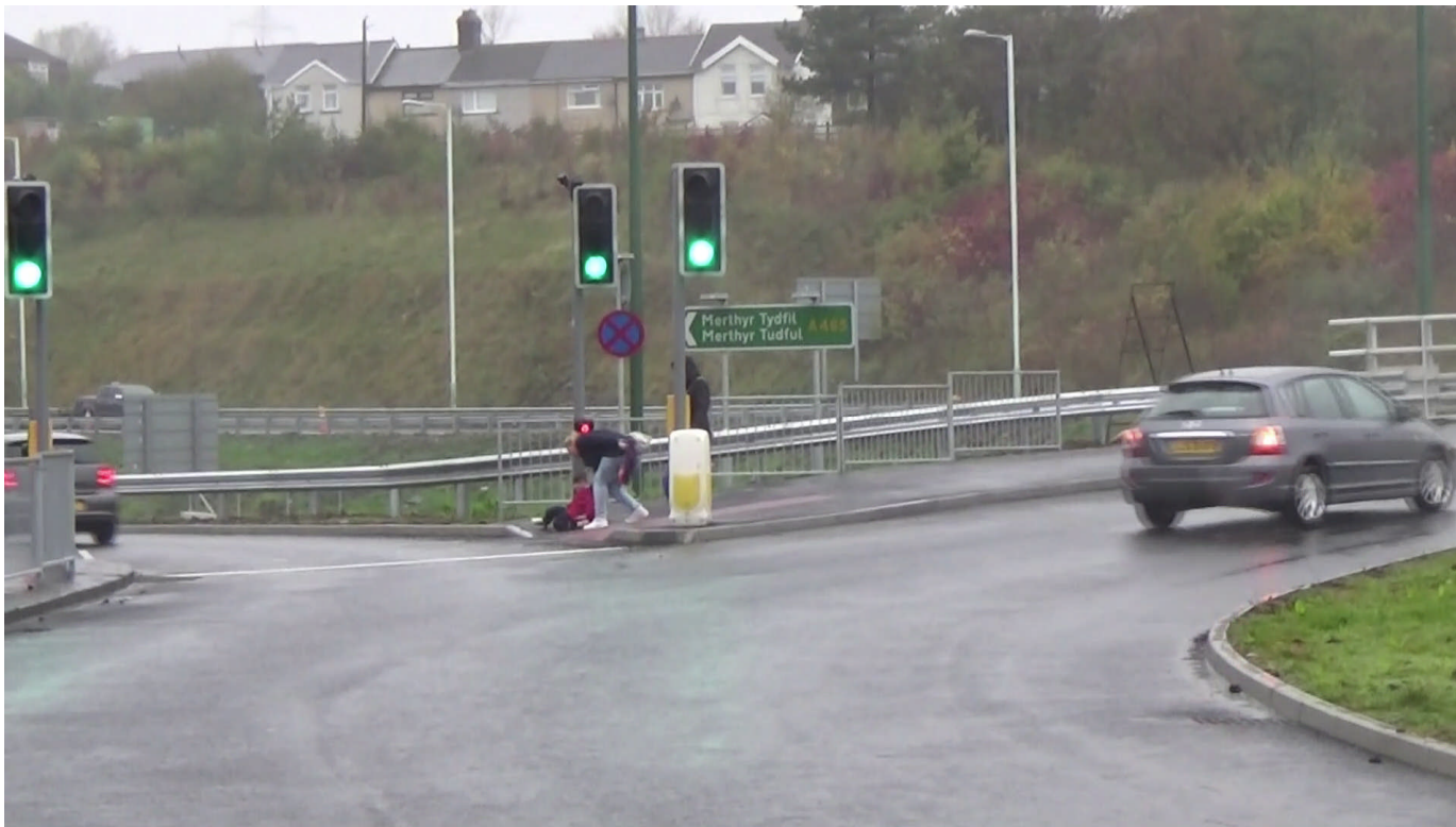
Figure 26 Child slips on wet tactile paving at on west-bound Section 3 on ramp of Nant-Y-Bwch roundabout just after car beyond accelerates of roundabout onto slip road.
